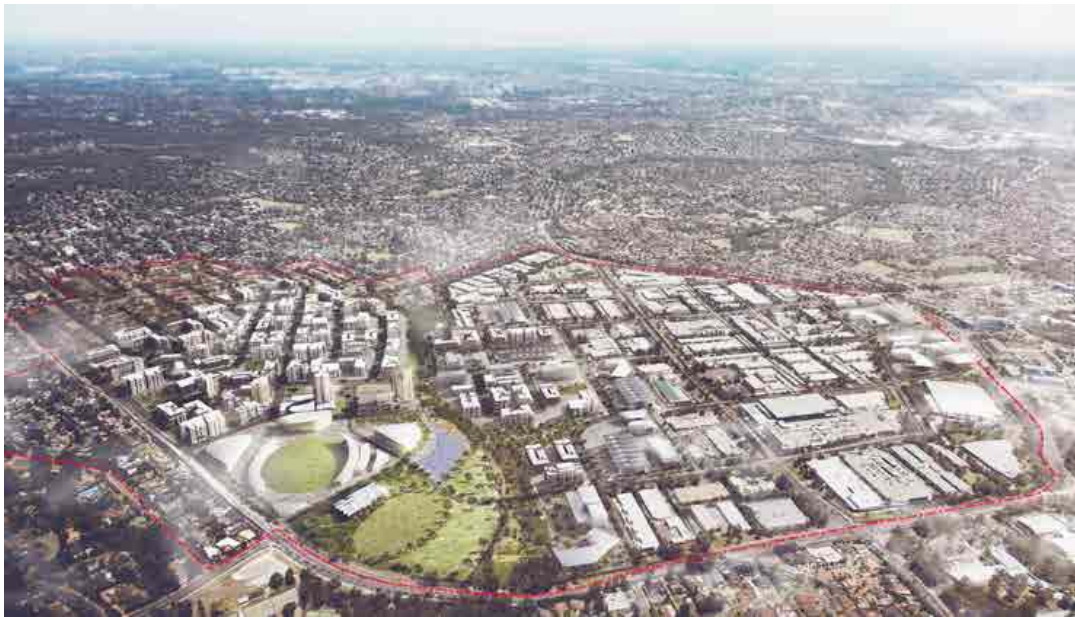
Figure 1 Aerial view of the envisioned Showground Station Precinct
